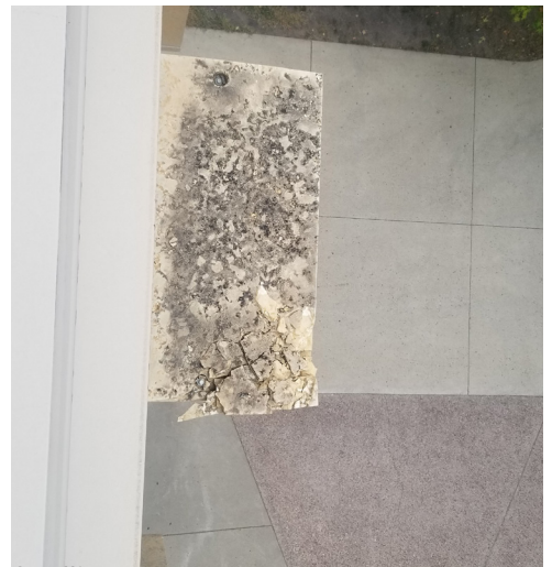
Spalling Limestone
