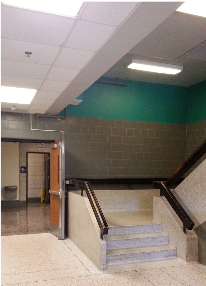
Typical Stair Landing in Armstrong Hall
