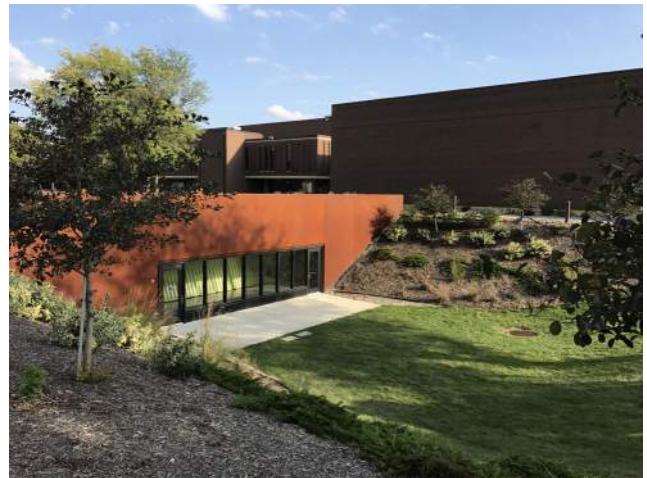
Figure 2.1-A. The campus Amphitheatre located between Memorial Library and the Centennial Student Union. The glass windows at the base are part of the tunnel connection between the library and student union.
